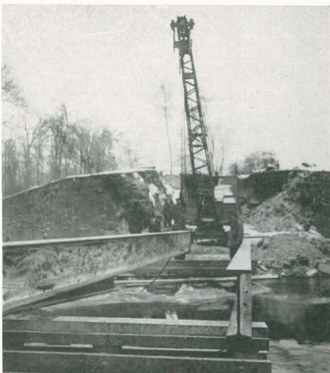
Placing steel stringers in place during the construction of a fixed bridge across the Saar River
