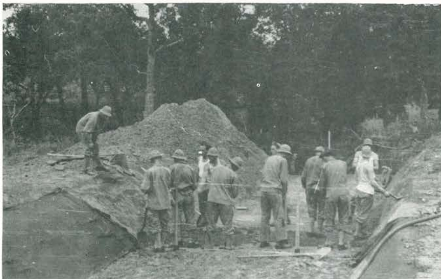
Camp Swift, Texas. 320th Engineers constructing spillway to dam using soil cement materials for surfacing of sides and bottom of spillway.
