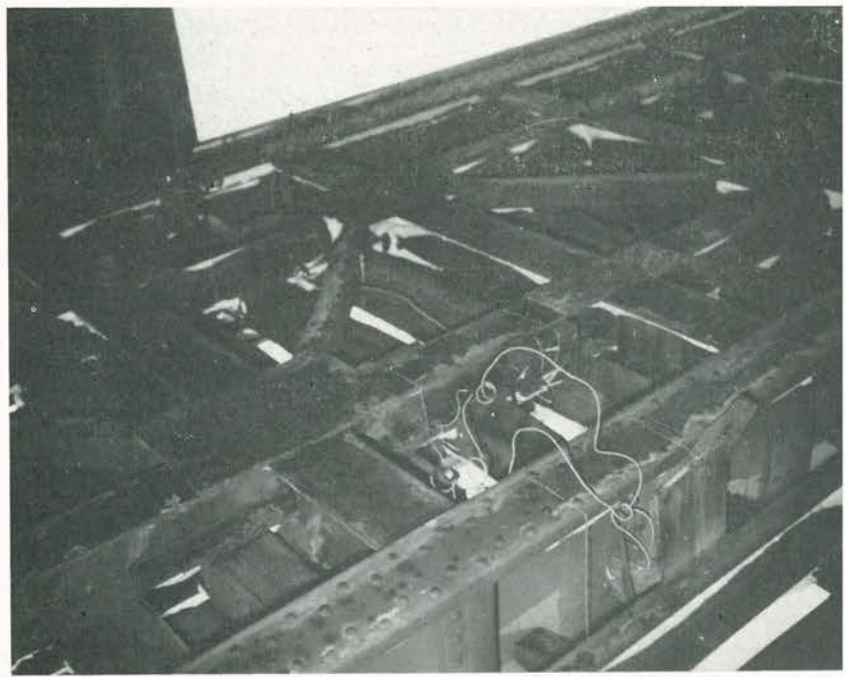
Railroad bridge prepared for demolition in defense plan. Picture shows detail wiring of charges
