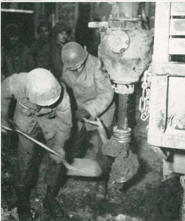
Private Jensen and Private First Class Carter of Company A cleaning blades of earth auger while preparing road crater in defense plan
