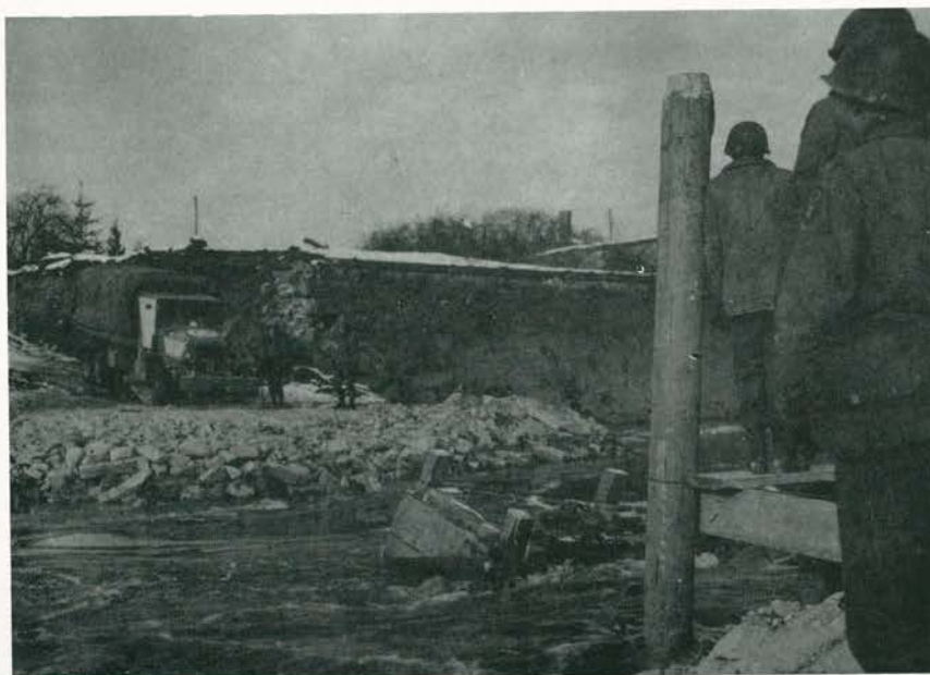
Using winch to pull crib into position at river crossing, Saarlautern
