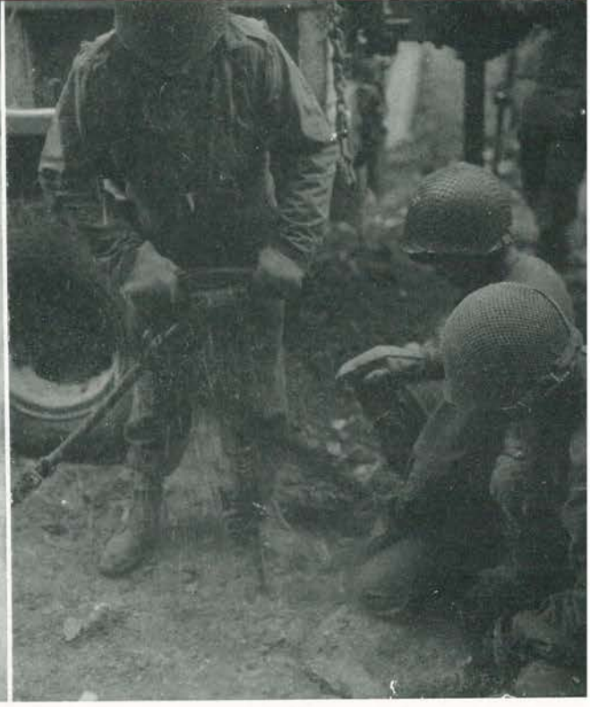
Breaking pavement prior to digging holes for road crater in defense plan. Corporals Dubois, Lepsey and Private Jensen of Company A
