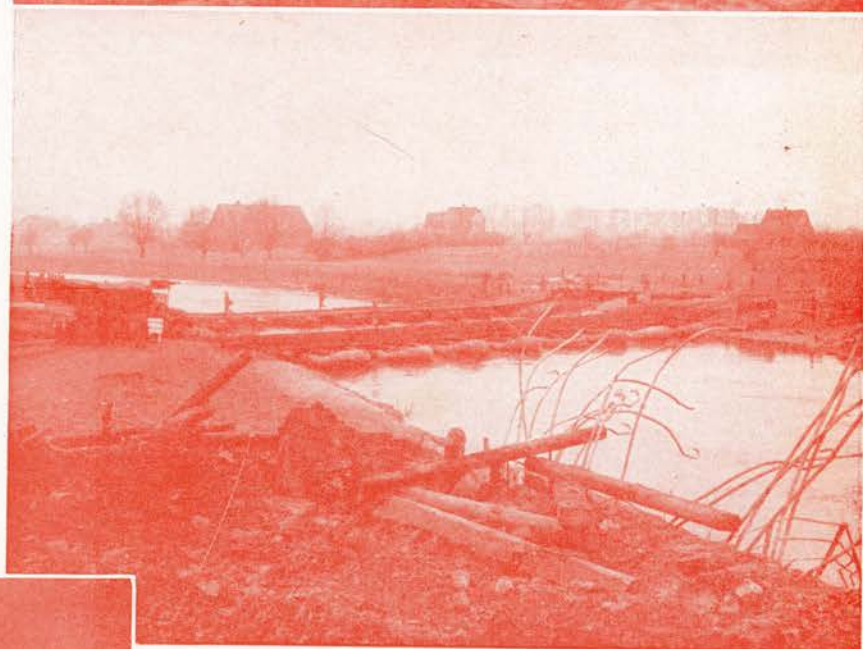
Floating treadway and pon- toon bridges constructed by Company C across Lippe River
