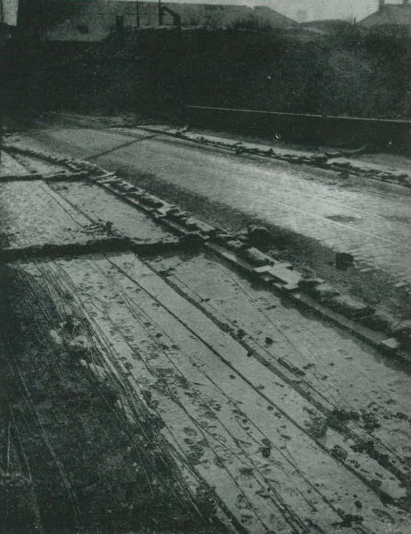
During Battle of Bulge the bridge across Saar River at Saarlautern, Germany, was prepared for demolition by 320th Engineers. Demolition wires protected by planking and sandbags. January, 1945
