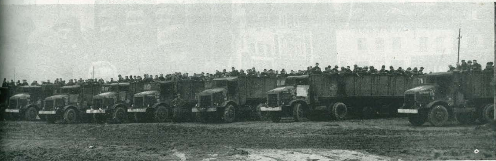
. . . and piling into waiting trucks
