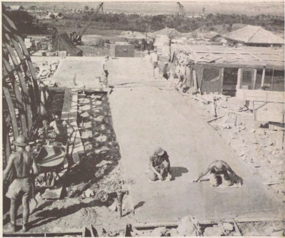
Finishing Concrete Slab for Reefers
