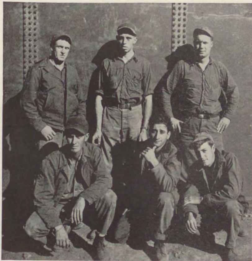
Tank Testing Crew
