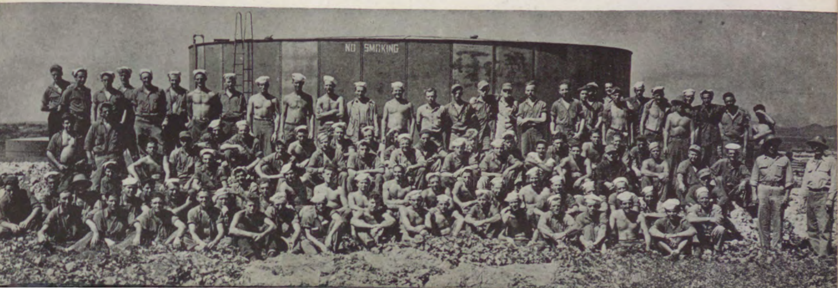
Tank Erection Crews
