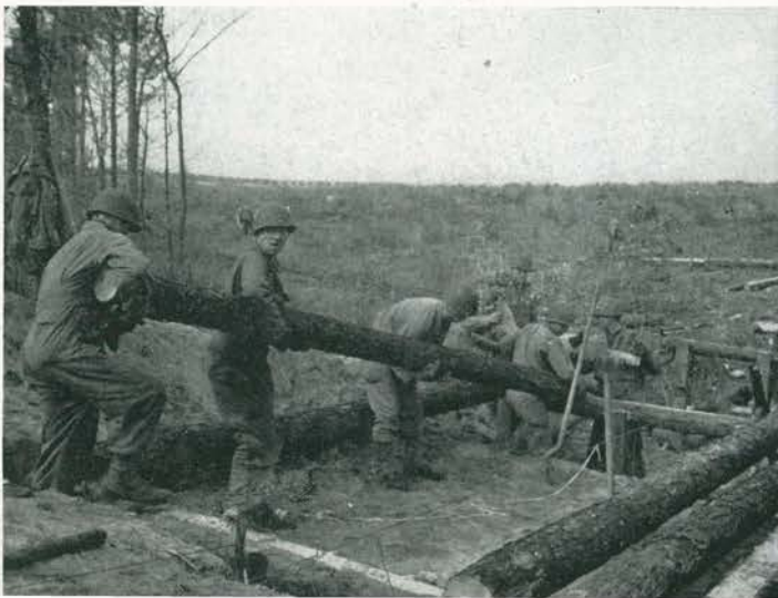
Laying Stringers for first bridge constructed by Co. A— During Training
