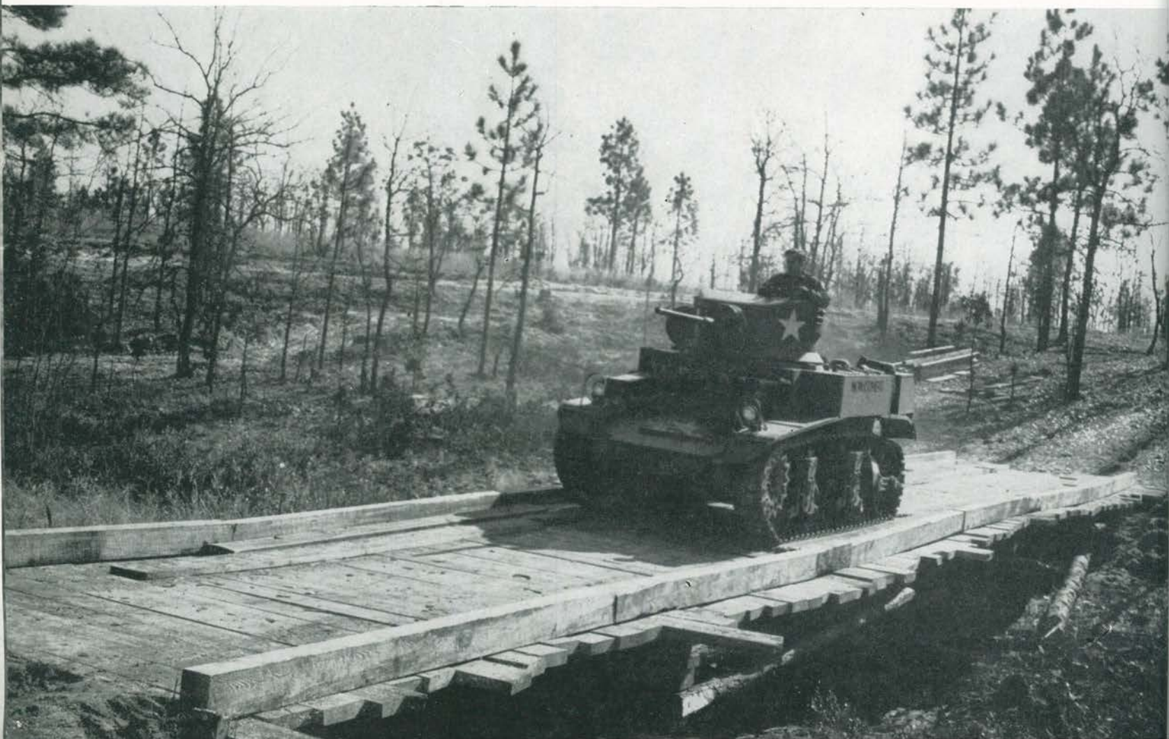
Completed fixed bridge built in basic training, tank weight, approximately 13 tons
