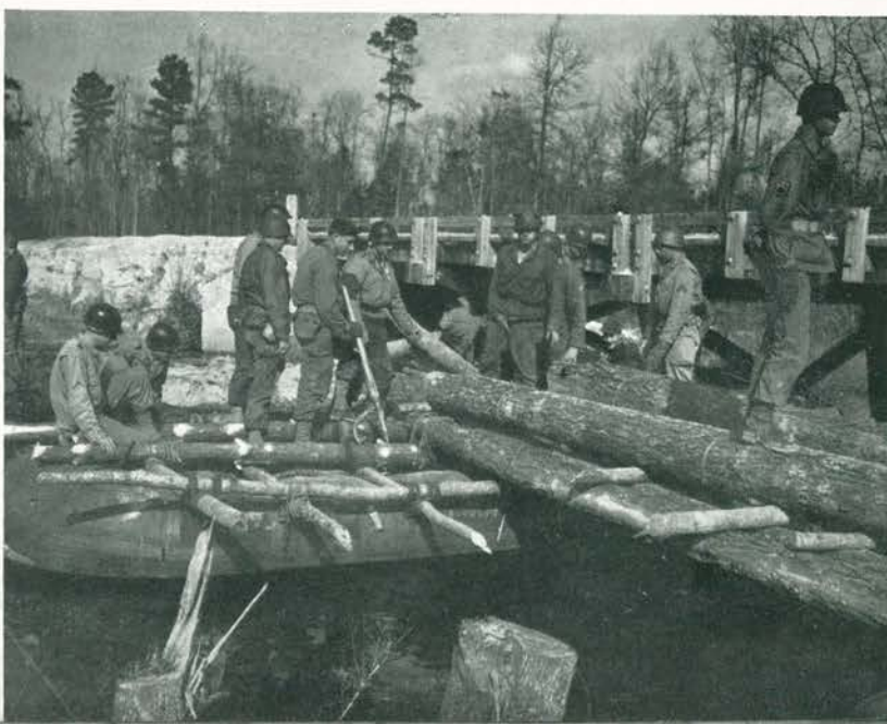
S/Sgt. Knebllick Supervising placement of stringers from shore to Ponton
