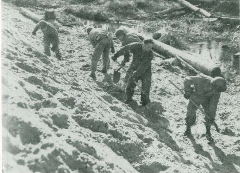
Company A—Constructing the approach to an expedient Ponton Bridge, to cross Downing Creek
