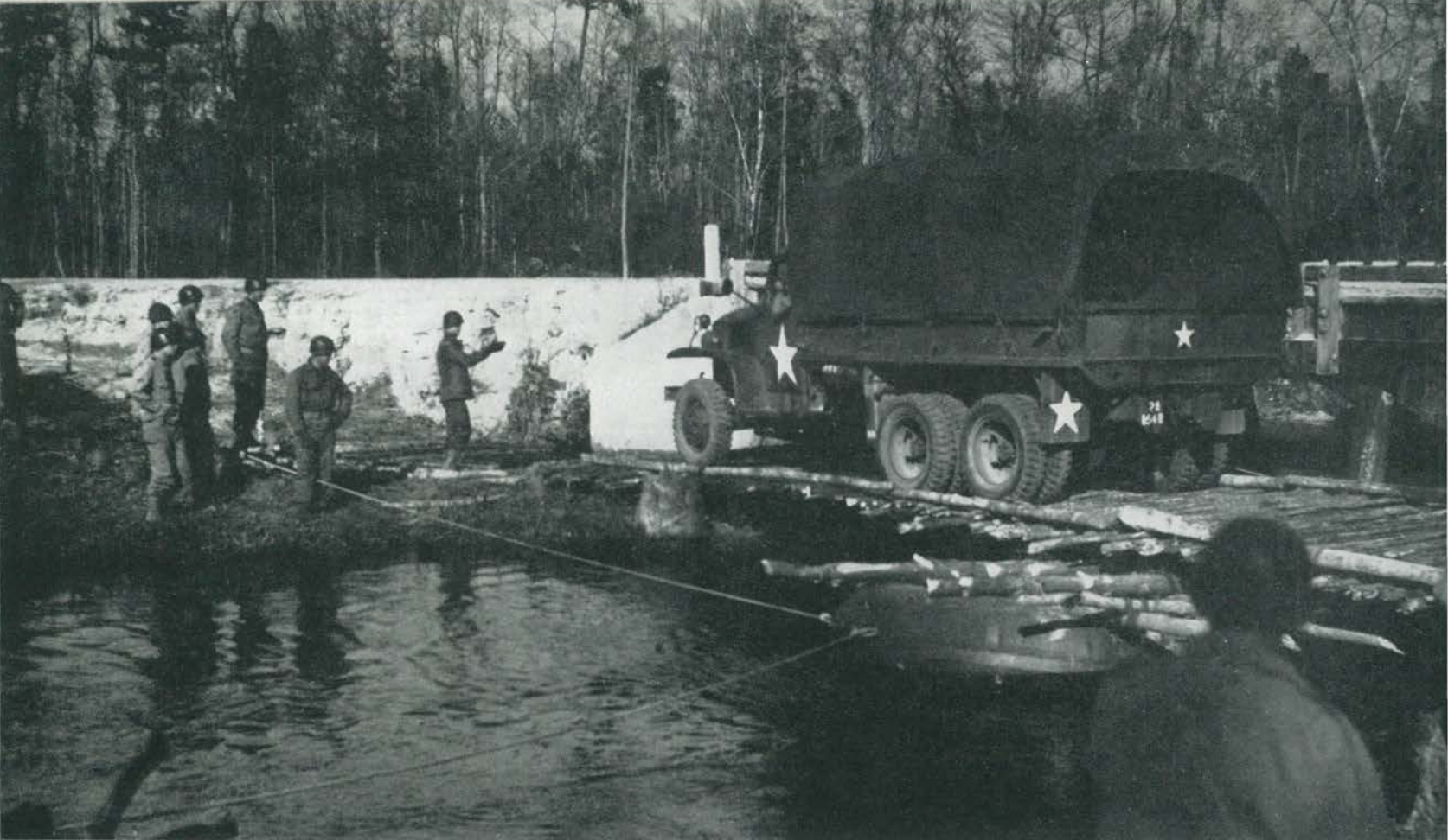
Completed Ponton Bridge open for all division traffic. Bridge was completed in less than three hours, capacity of 15 tons
