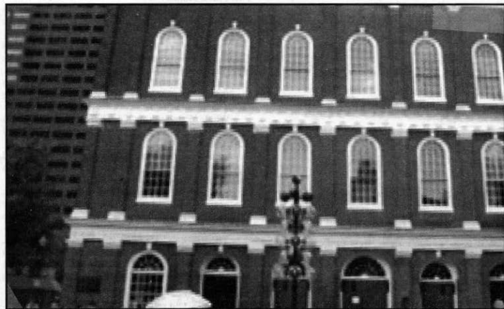
OLD FARNEUIL HALL MARKETPLACE BUILDING
