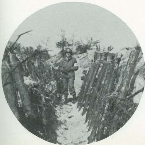
Trench—Frankfurt Race Track
