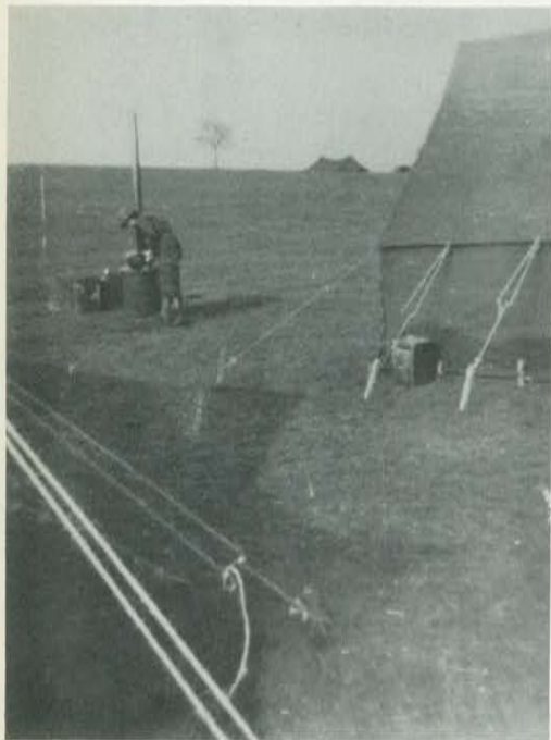
Hot water supply
