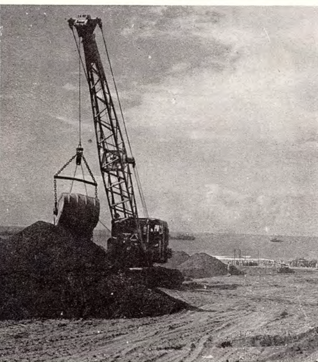
Dragline Digging Drainage Ditch.
