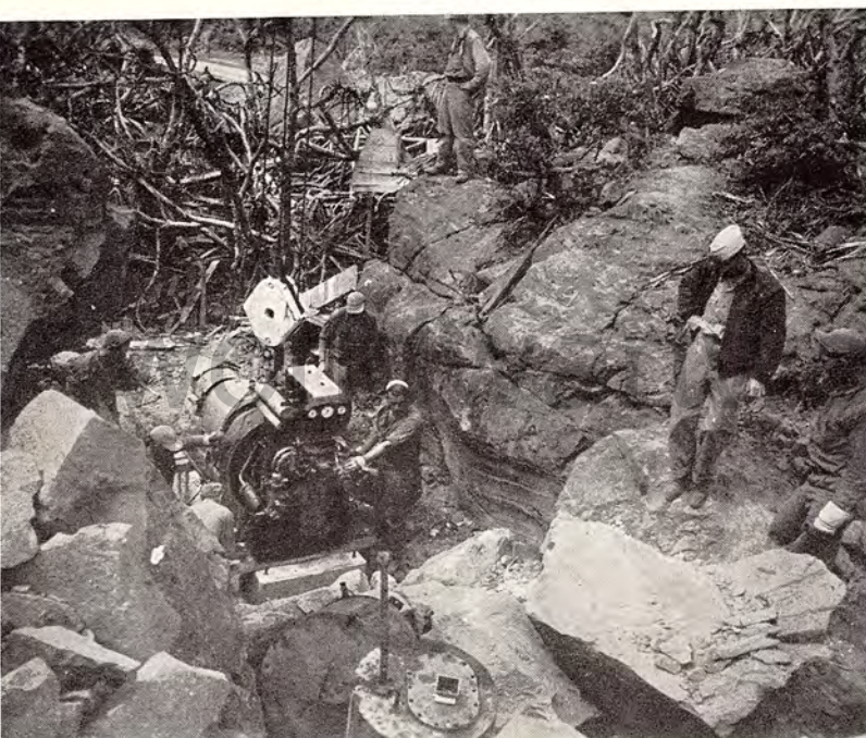
Installing a Jap Generator.
