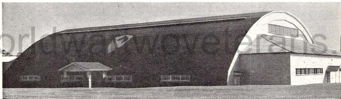
Named in honor of Captain William C. Cornelius, killed in the division's campaign in the Admiralties, the field house at Camp Drake serves as a sport center for the command post. It is also the scene of many division-final indoor sports events.
