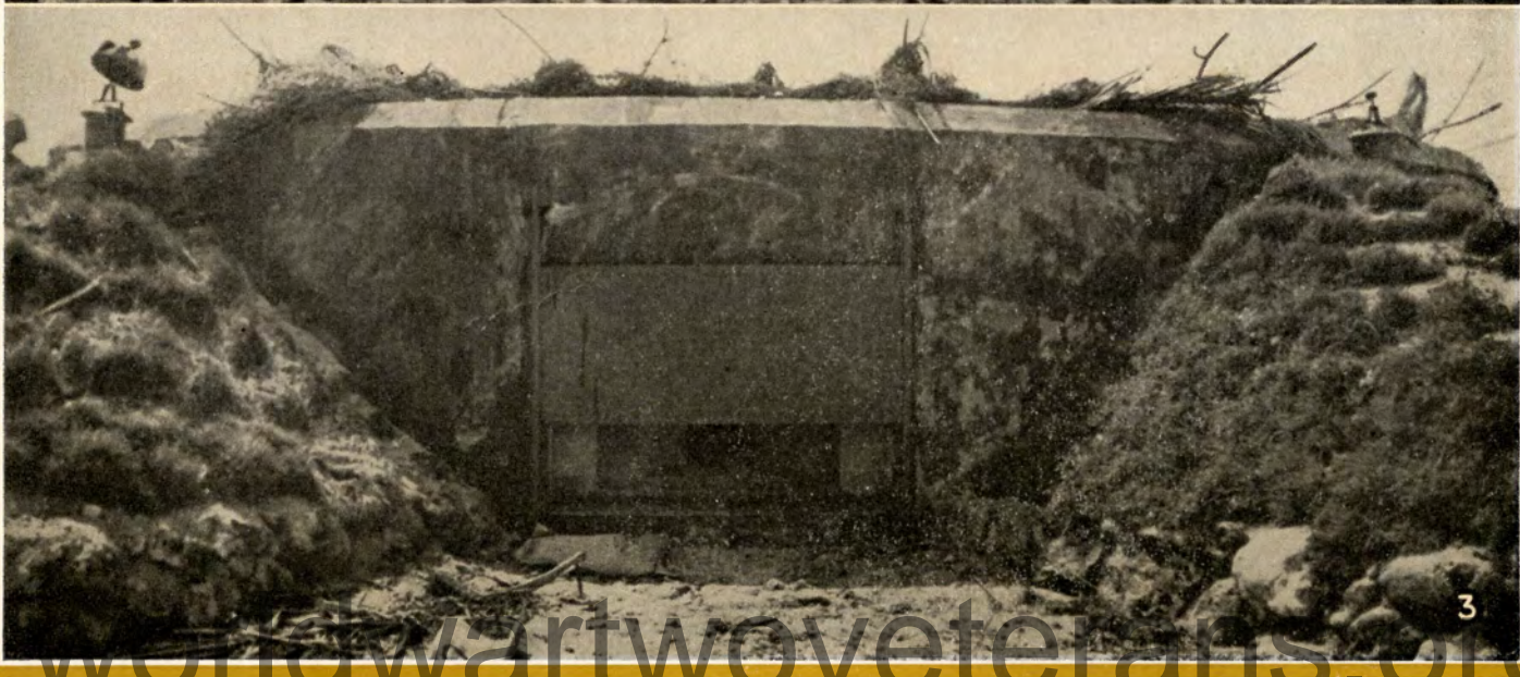
1-Twisted wreckage was all that remained of the pier on Namur after the naval bombardment. 2-This massive, German-type blockhouse, guarding the beaches, was destroyed by our naval gun fire. 3-Another blockhouse, with walls four feet thick and gun apertures covered by sliding steel panels, was captured in the attack.
