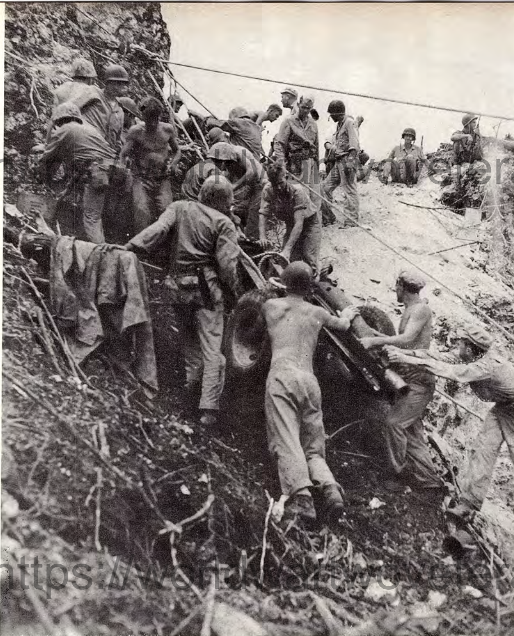
BLOCK AND TACKLE: Artillerymen hoist a pack howitzer to a ridge top at Umurbrogol
