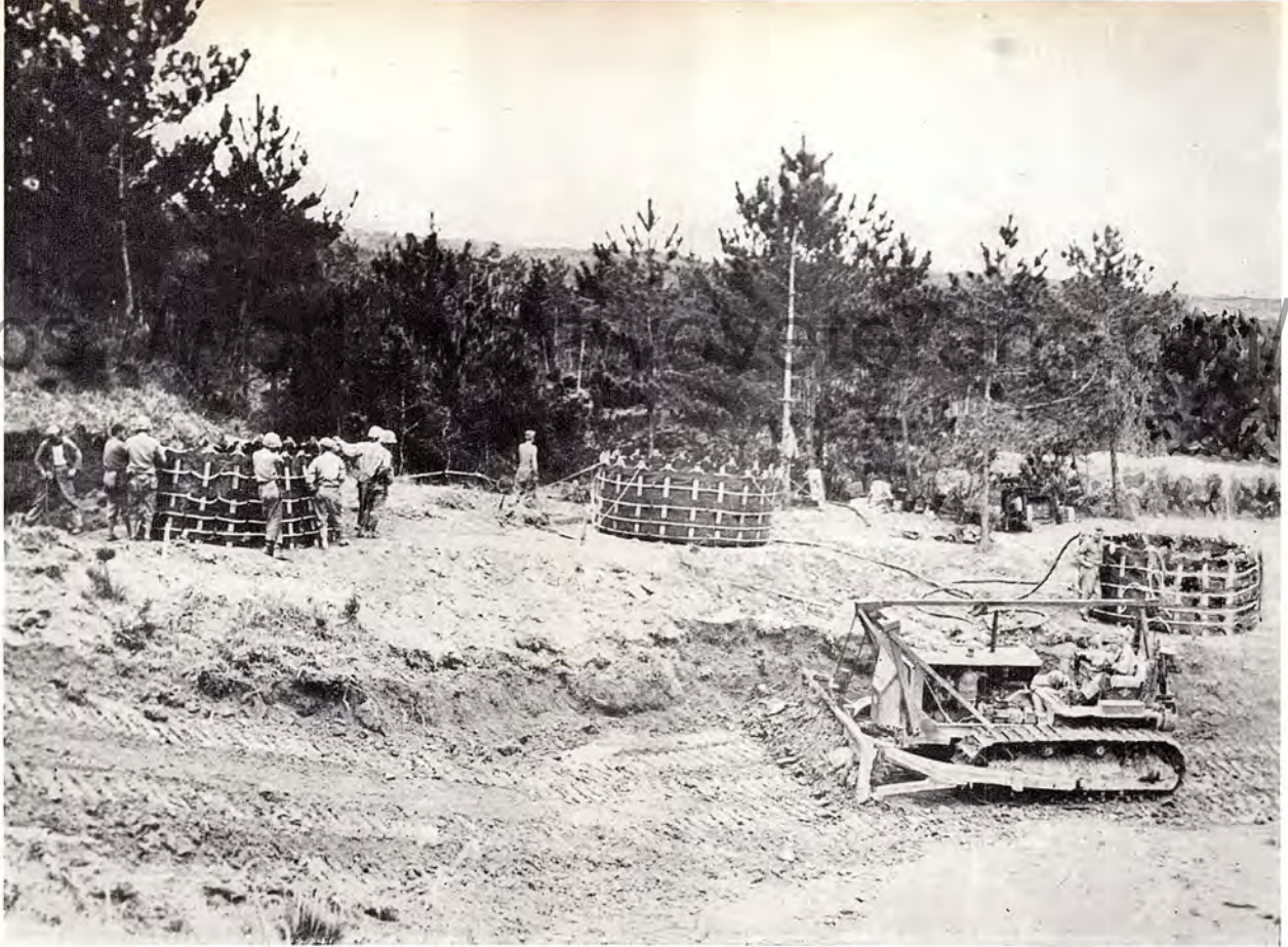
WATER POINT: Collapsible water tanks on Okinawa, erected by the engineers
