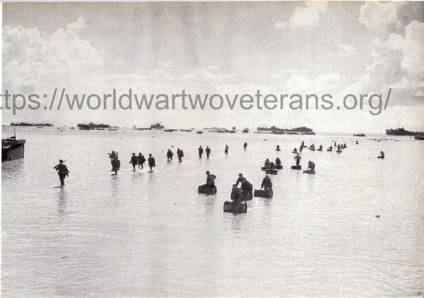
SUPPLIES ROLL IN: Drums of gasoline and water are rolled across the 500-yard reef from the landing craft which unloaded them at the seaward edge of the reef
