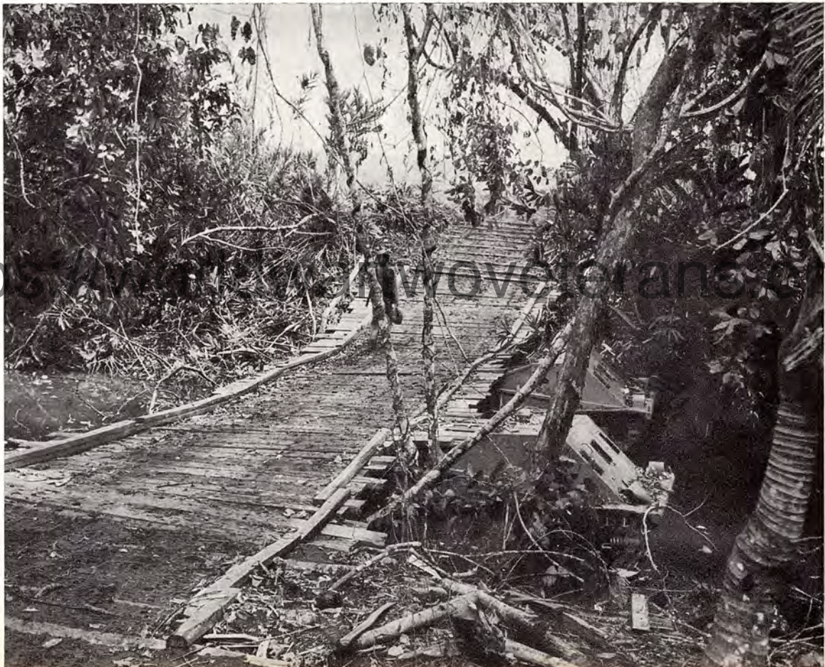
BACKWATER BRIDGE: Engineers planned this bridge aboard ship, stole or "borrowed" the lumber from ships' stores and were ready with amtracs to make this improvised crossing of a brackish jungle stream
