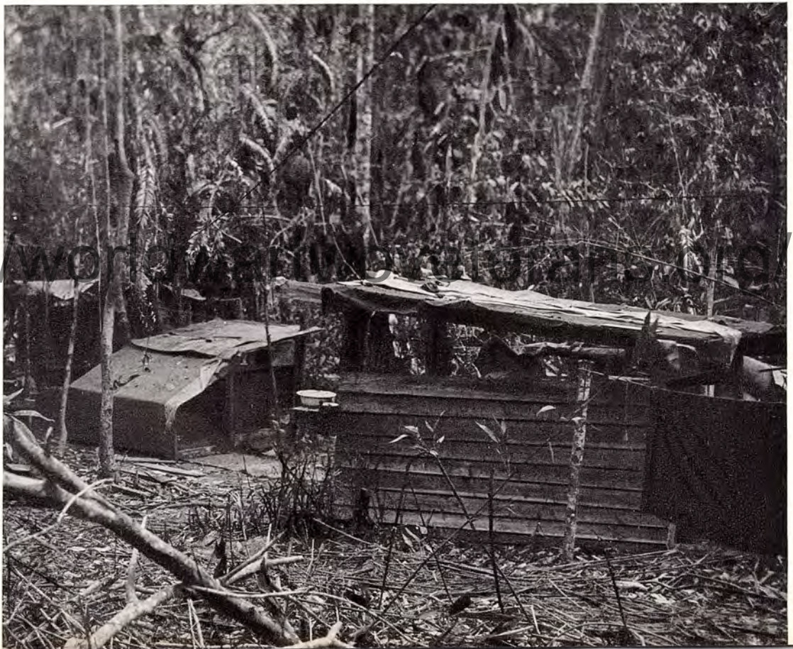
A LITTLE WOODEN SHACK: Here are typical Guadalcanal huts built when men settled down to the long haul of that campaign
