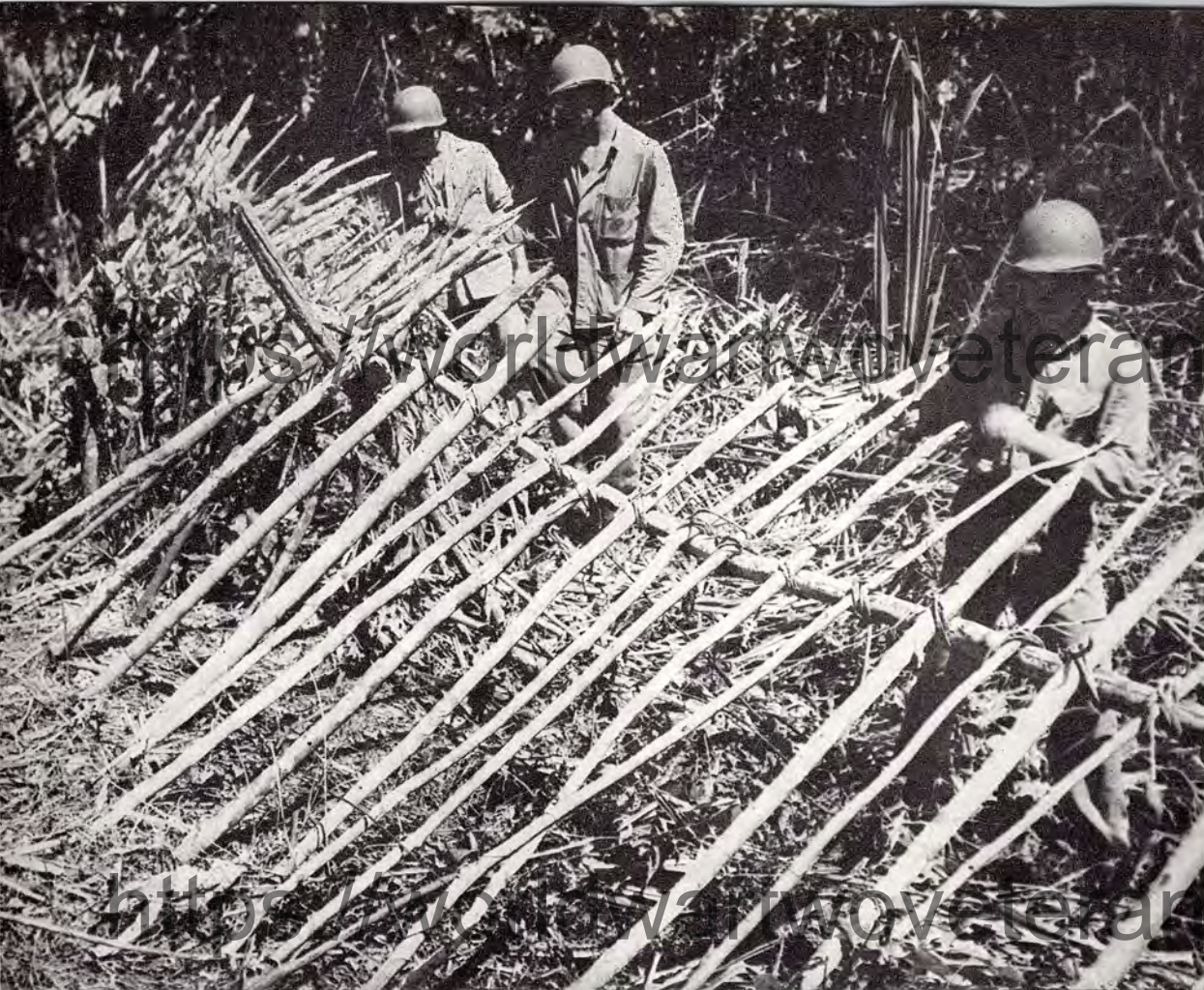
HASTY DEFENSE: Lacking barbed wire, Marines lash together sharpened stakes to protect their lines
