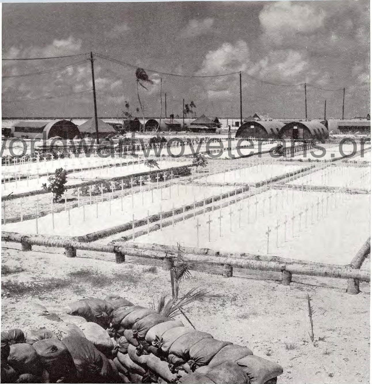
THE PERMANENT CEMETERY , in the same area as the battle cemetery, was decorated with shining coral and neat white crosses, and surrounded by a wall of coconut logs. Seabees did much of the work.
