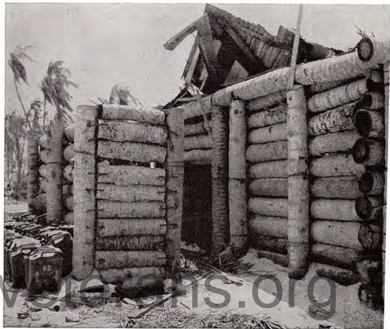
HOW JAPS BUILT Fortress Betio shows up clearly in this coconut blockhouse, which is reinforced with heavy steel.
