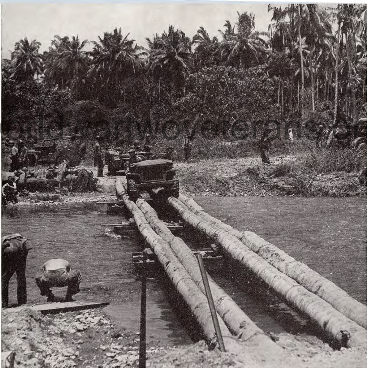
THE ATTACK PROGRESSES as jeeps roll across coconut log bridges ingeniously devised by the engineers, bringing ammunition, food and supplies to the front. This assault was successful and river was secured.
