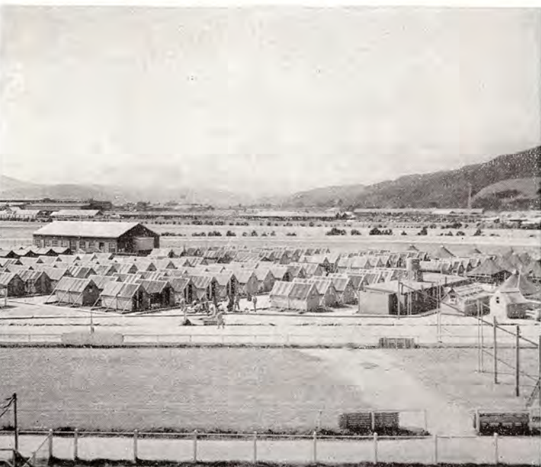
TYPICAL SHELTERS built for Second Division camps in New Zealand are these enlisted men's huts— at last after incredible travail.
