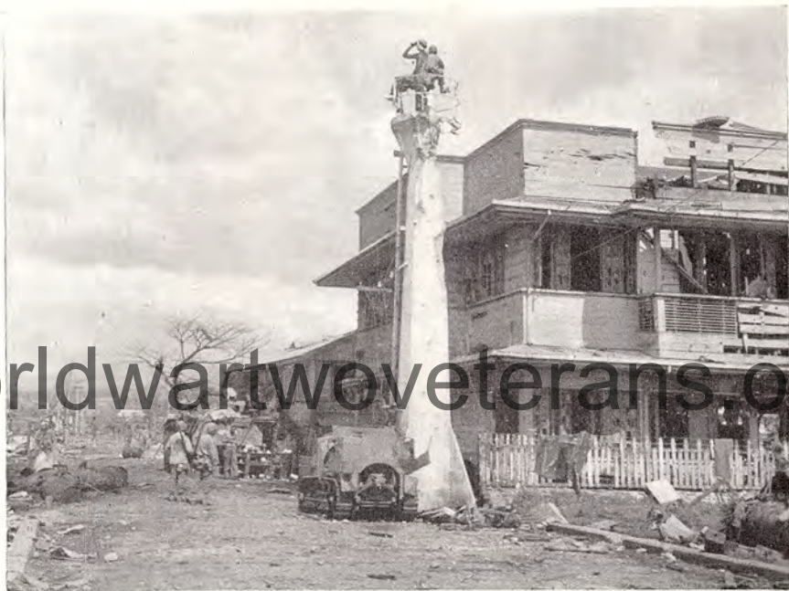
Antiaircraft observation tower near the pier at Ormoc.
