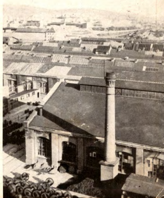
Corner: Locomotive back shop, Esslingen
