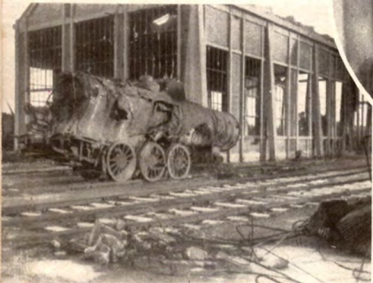
Above: A big repair job—Aulnoye enginehouse
