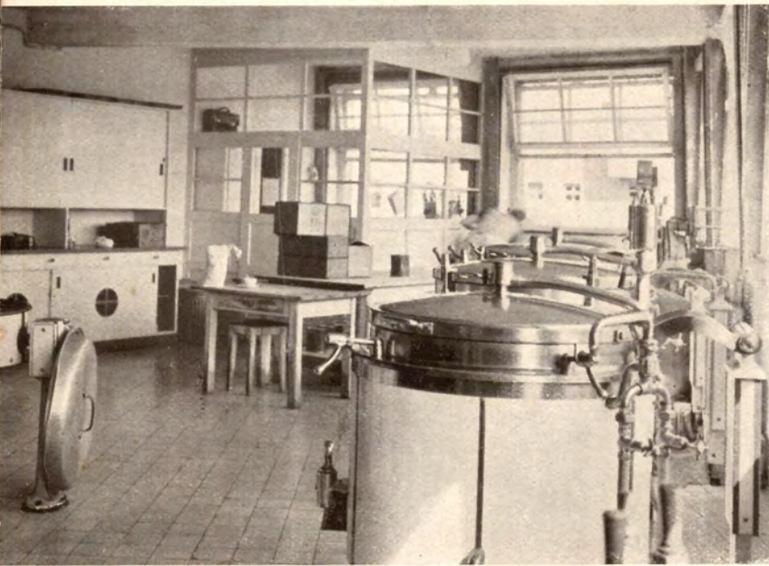
Above: Modern kitchen, Esslingen mess hall
