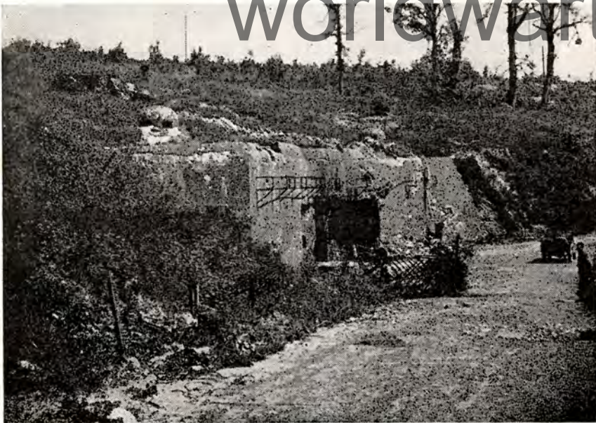
Supply entrance to Ft. Schiesseck. Small railway cars could roll right into the fort. Note steel cupola on top.
