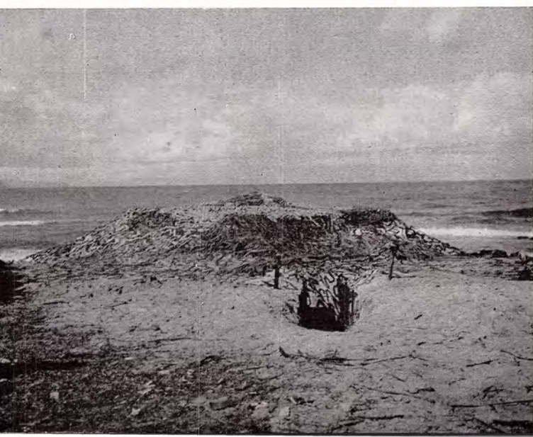
Well camouflaged beach machine gun pill box. These were installed and manned all over the islands.
