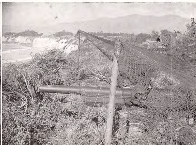
Another emplacement near Santa Barbara
