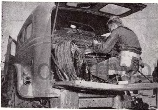
Signal Company tackles problem of wire laying.
