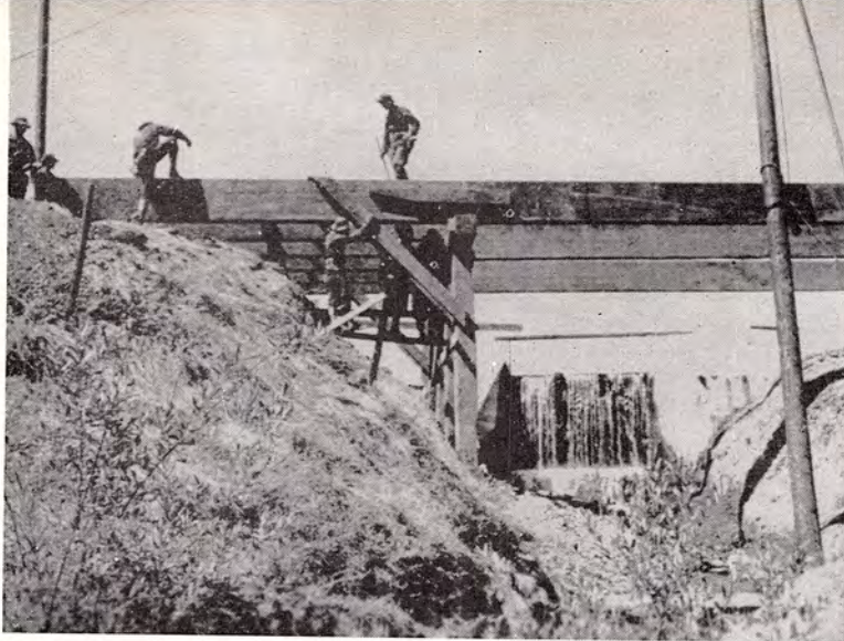
The Engineers Erect a Bridge
