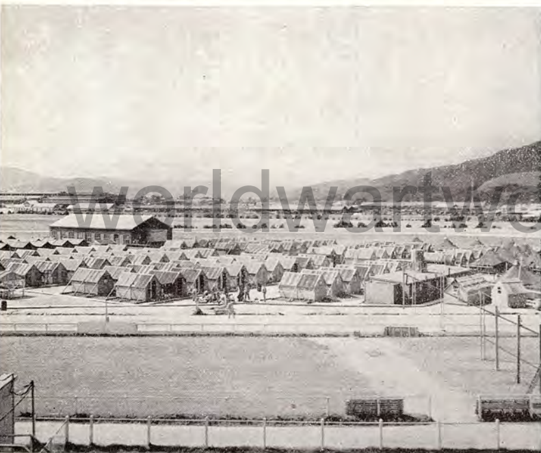
TYPICAL SHELTERS built for Second Division camps in New Zealand are these enlisted men's huts.
