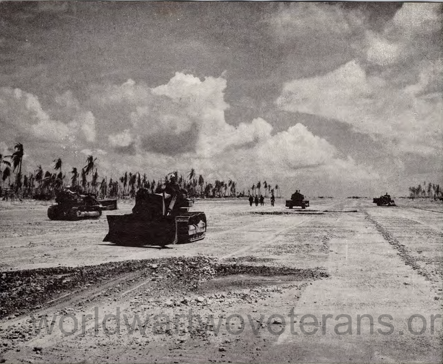
BEFORE BATTLE ENDED , the Seabees had their bulldozers ashore and were beginning to level and grade the airstrip that was renamed "Hawkins Field."
