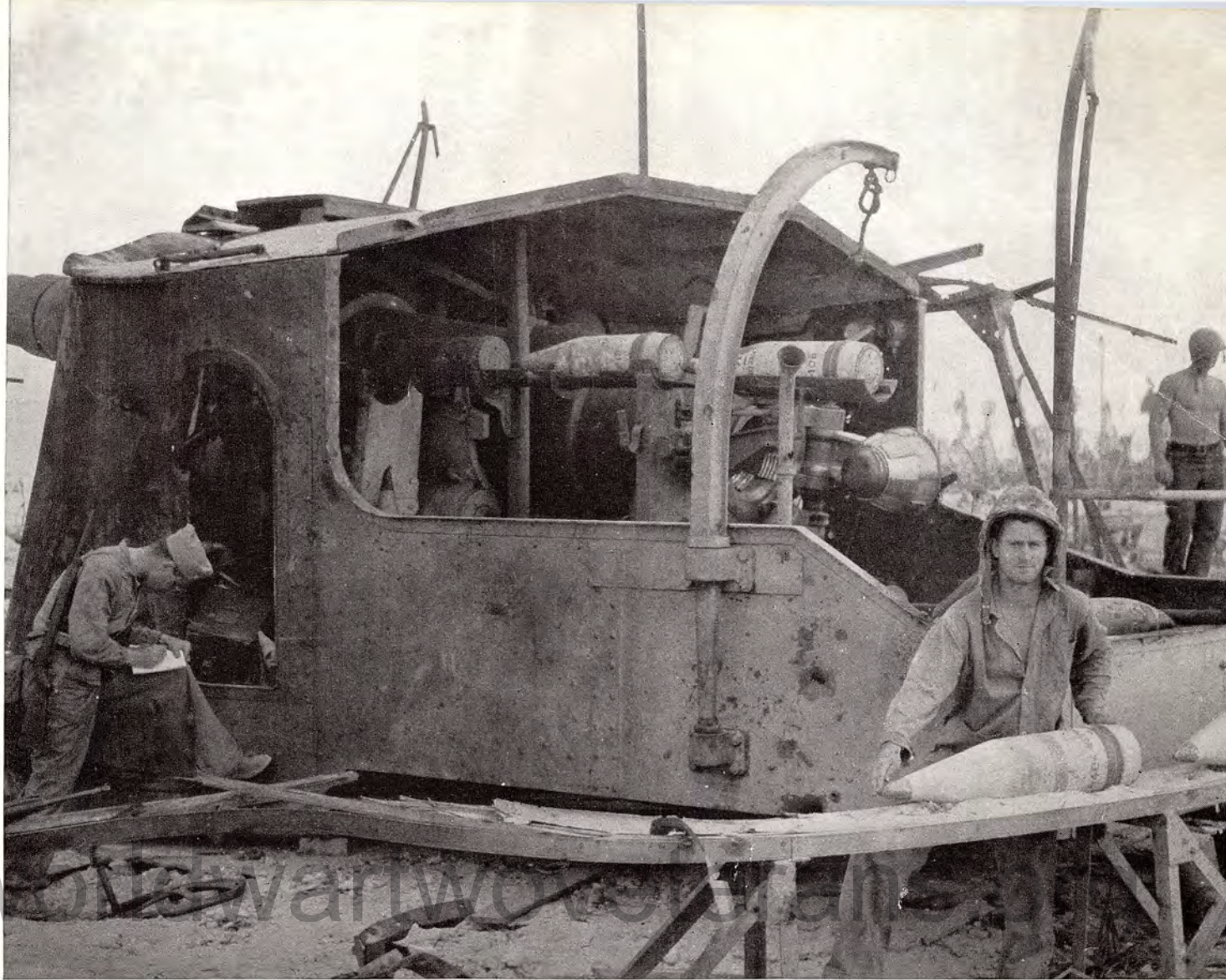
JAP BIG GUNS on Betio were fed by this circular track, which kept the 8-inch shells moving toward breech. Here Marines take notes on the mechanism soon after the end of the battle.
