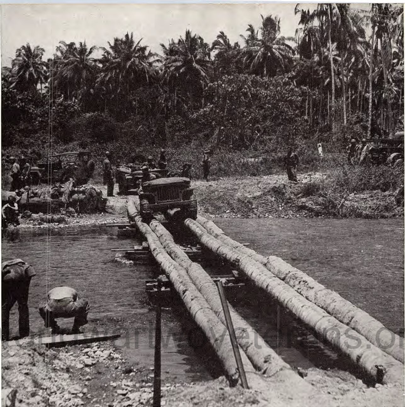
THE ATTACK PROGRESSES as jeeps roll across coconut log bridges ingeniously devised by the engineers, bringing ammunition, food and supplies to the front. This assault was successful and river was secured.
