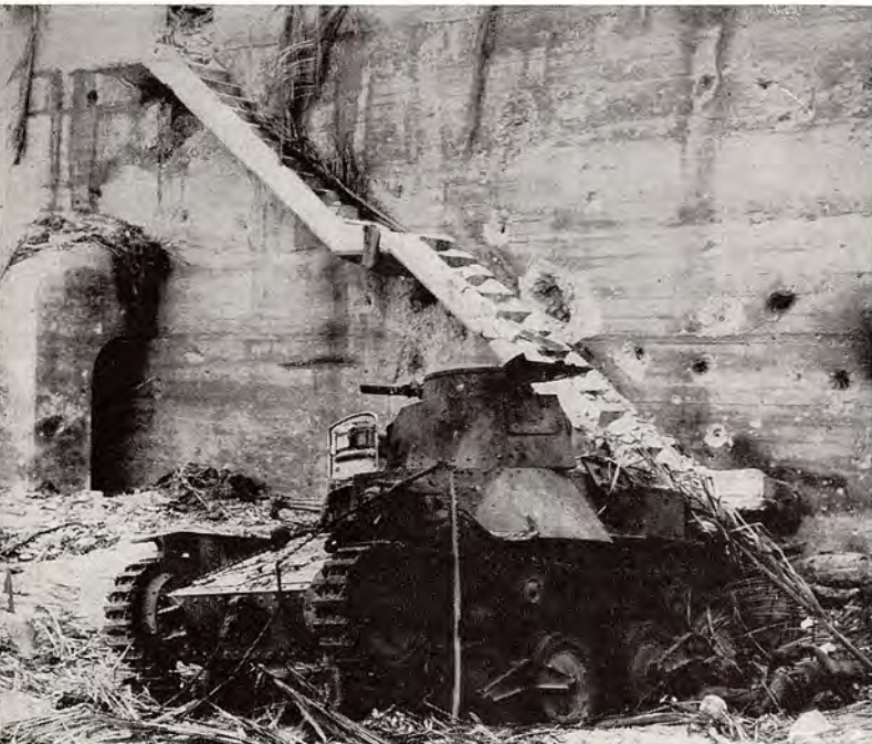
THE JAP COMMAND POST on Betio was built of concrete reinforced by steel. A disabled Jap tank is in foreground.
