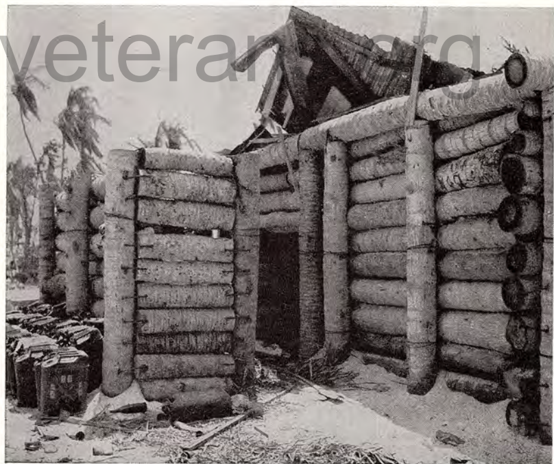
HOW JAPS BUILT Fortress Betio shows up clearly in this coconut blockhouse, which is reinforced with heavy steel.
