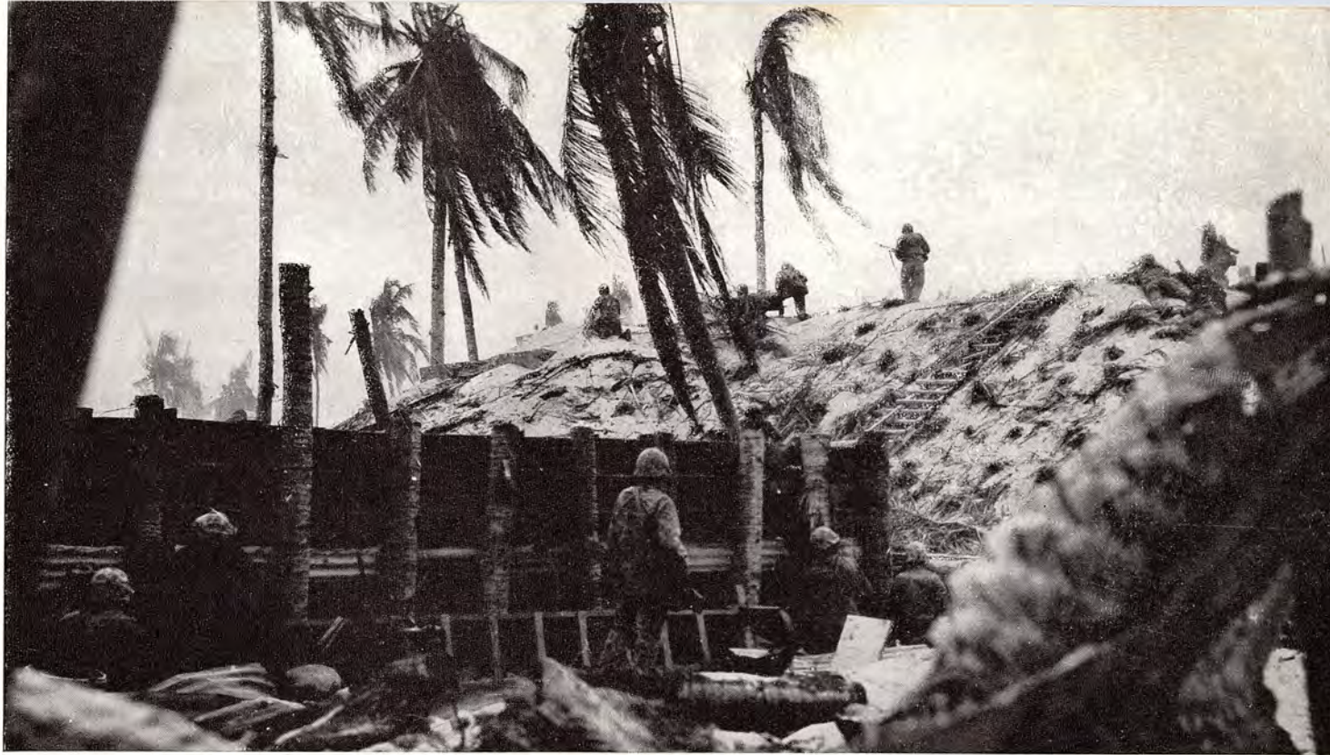
CREST OF BOMBPROOF is reached by Marine attackers. Assault demolition personnel used ventilating ports to burn out the interior of the power plant. Several Jap counterattacks were repulsed.
