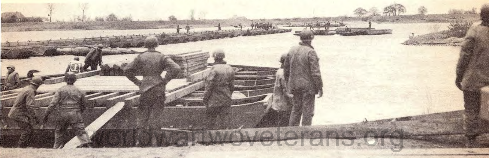
Engineers were shelled mercilessly as they built the pontoon bridge across the Elbe but they succeeded as always,
