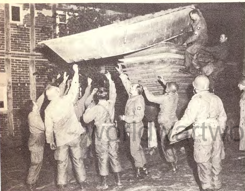
Above—The "Recons." were briefed for the initial crossing. They handled their own assault boats in the absence of Engineers. Our Regiments were still on their way from the Rhineland.
