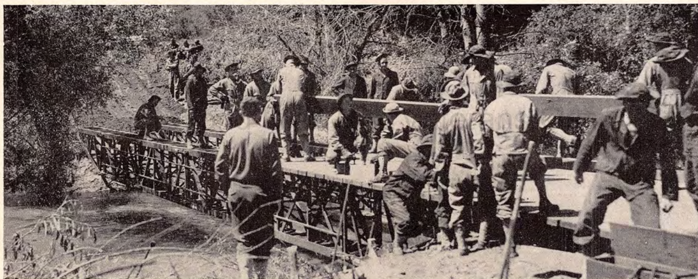
The 116th Engineers build a bridge over the San Antonio River at Hunter Liggett.
