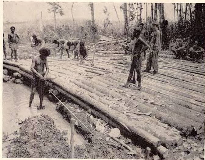
Natives construct a culvert on a new all-weather road somewhere in New Guinea.
