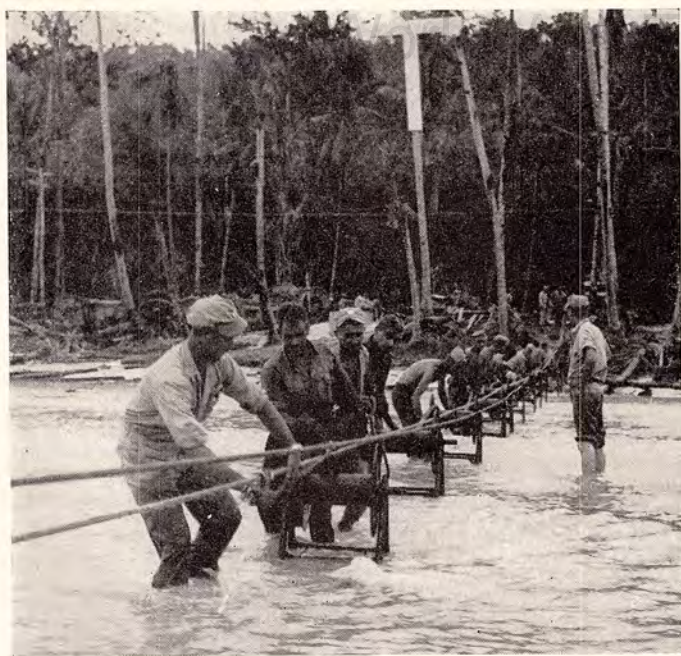
Men of a signal company lay a submarine cable from Biak to Owi Island.
