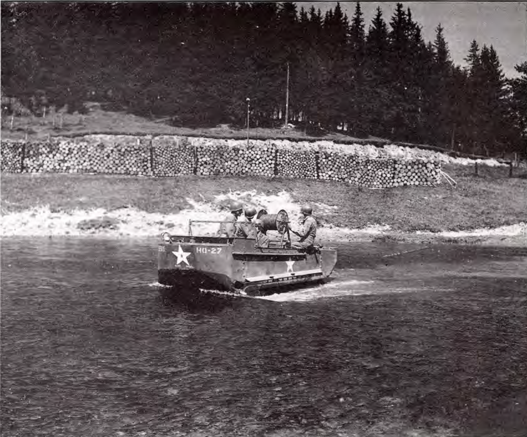
Wire-laying weasel used by both infantry and artillery battalions for use both on water and land.
