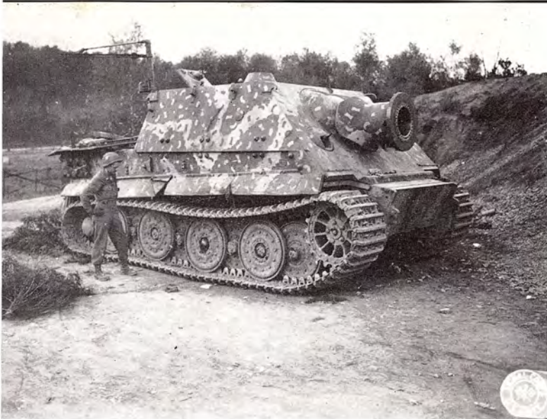
Short barrelled heavy rocket projector mounted on tiger tank captured near Menden, Germany.
