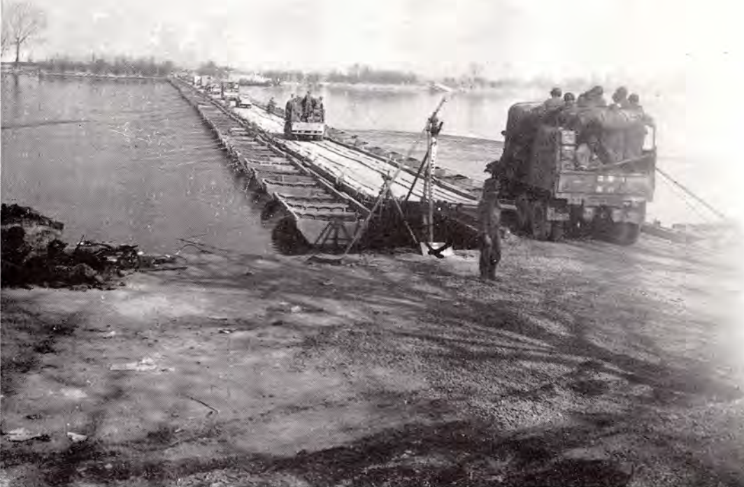
5th Division trucks cross Rhine River on ponton bridge that was built in half a day by Third Army engineers.
