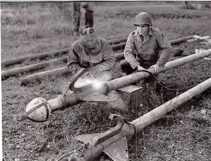
Tec. 4 Daniel O. Polte welds nose on "explosive snake" for use in assault against Fort Driant.
