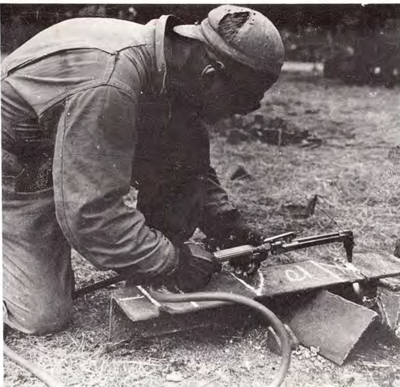
Welder is shown cutting piece of steel prior to making hedgerow cutter to place on 735th battalion tank.
