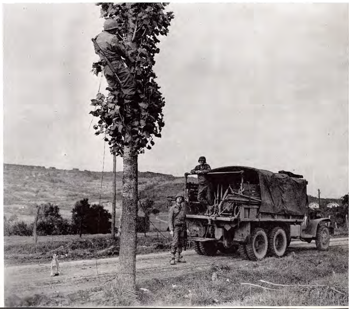
Fifth Signal Company wire construction crew fixes an overhead installation near Pagny, France.
