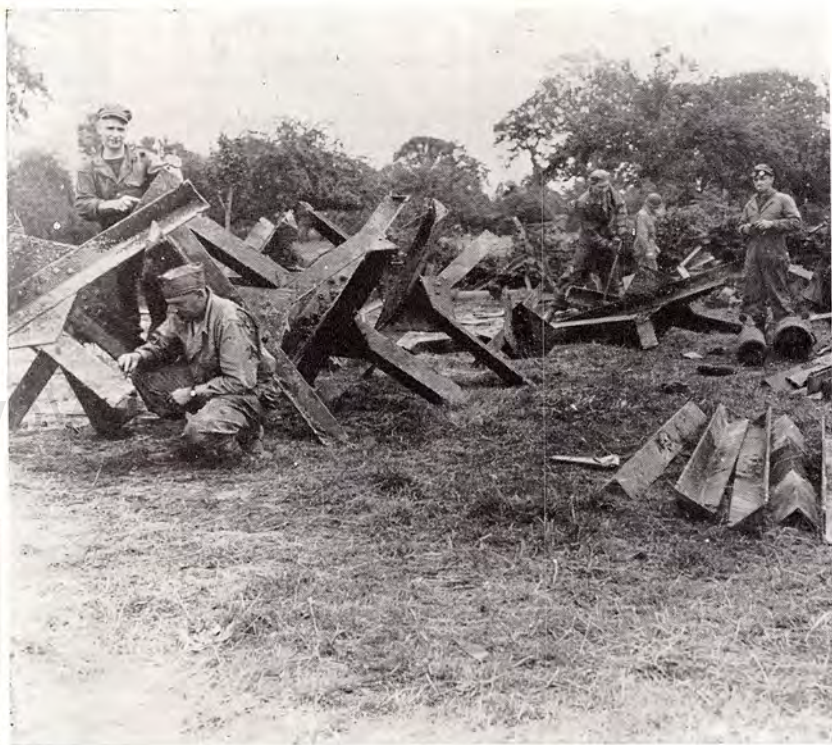
View showing hedgerow cutters being constructed for use on the front of tanks.
