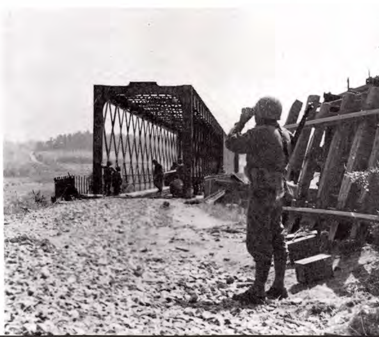
Engineers ready a railroad bridge in the Angers area to handle tank traffic.
