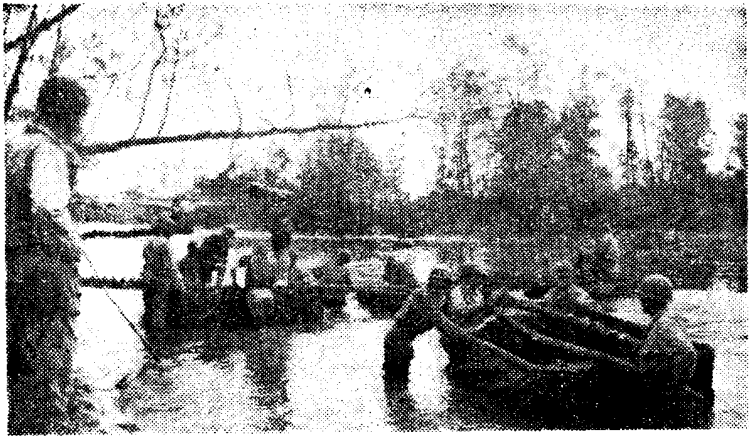
CROSSING RIVERS ON TENTS is child's play to men of 263d Engr. Combat Bn., as they demonstrate in pictures on this page. Above is scene of a stream crossing expedient class of an A & P platoon. Logs are being used to strengthen tarpaulins from GI trucks to be used as bridge pantoons.
