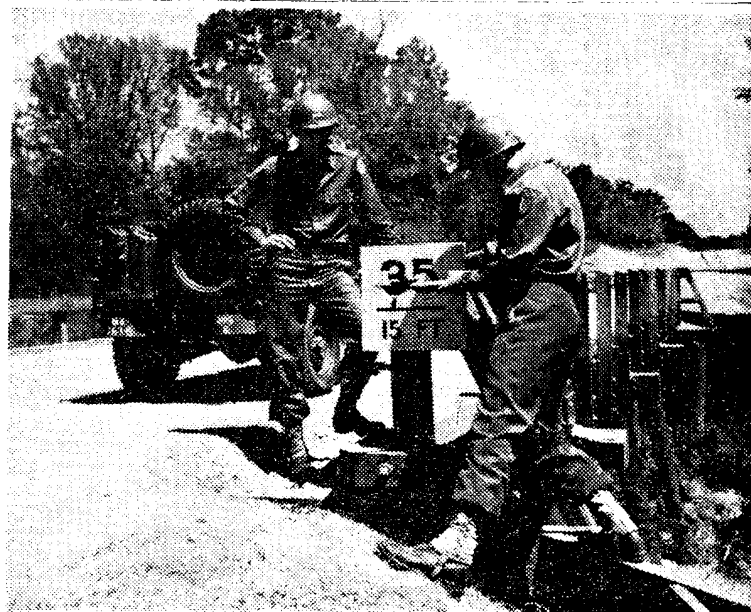
OVERLOADING of bridges within the Camp Van Dorn area should be eliminated by the new method of marking and classification completed this week. Classification of the bridges was accomplished by members of the S-2 section of the 263d Engrs., while signs similar to that depicted above were posted by the reconnaissance section of the same outfit.
