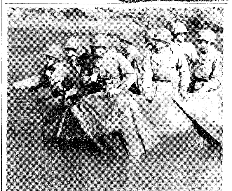
RUB-A-DUB-DUB, nine men in a tub . . . and men of 263d Engineers are ferried across a rapid stream, in ferry made from truck tarpaulin and boughs. The men built the ferry, then rode in it. Displacement and buoyancy of air are the secrets of this means of transportation. See page 7 for photos of how jeeps get ferried in the same way.
