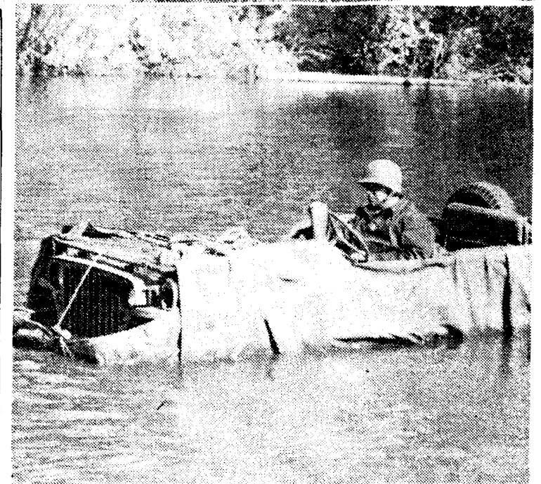
OOPSIE DAISY it's a new version of the seagoin' jeep, 2633d Engineers have rigged a river-crossing ferry from some handy boughs and a truck tarpaulin, and in top photo they're setting out to construct the "ferry" around a jeep needed across river. Bottom photo shows the driver, seemingly crossing the river with the current.
