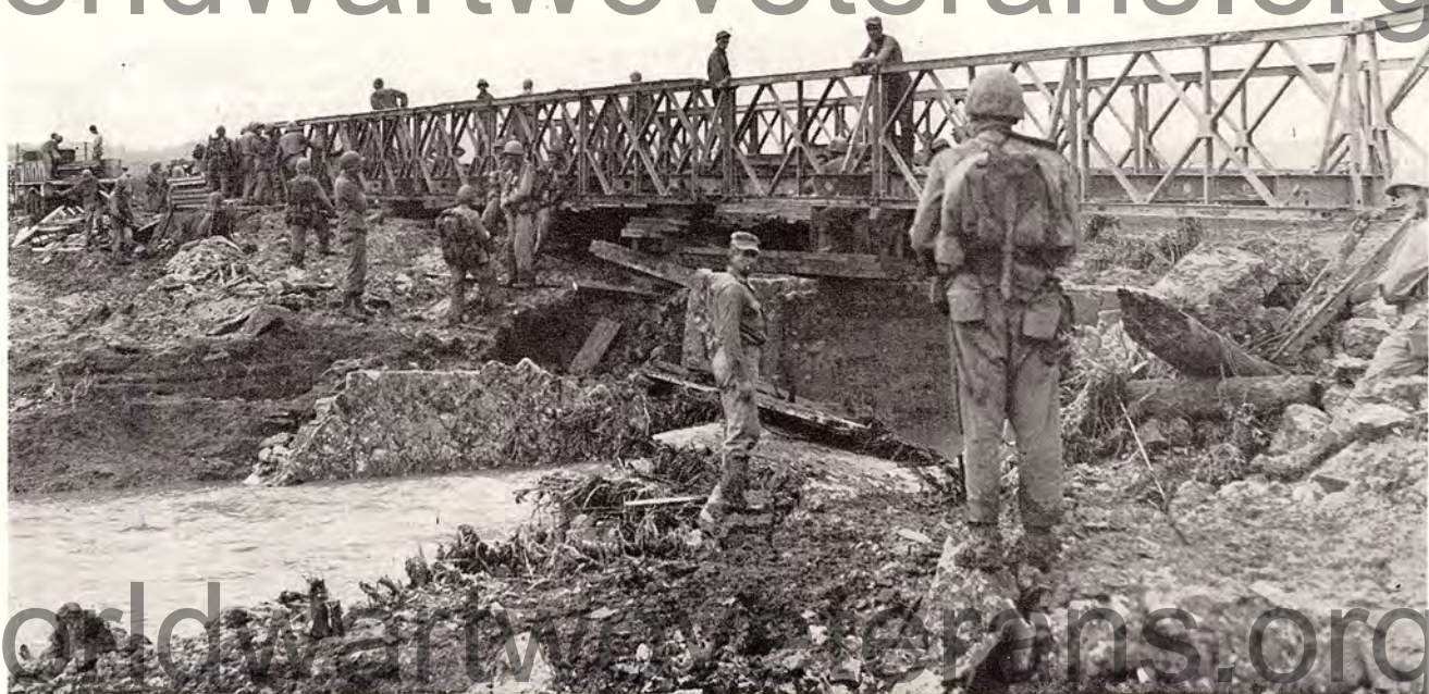
Top: Portable footbridge thrown across the Asato River by troops of the 6th Engineer Battalion. Bottom: The first Bailey bridge to span the Asato—erected under fire to permit tanks to join in the attack to the south.
